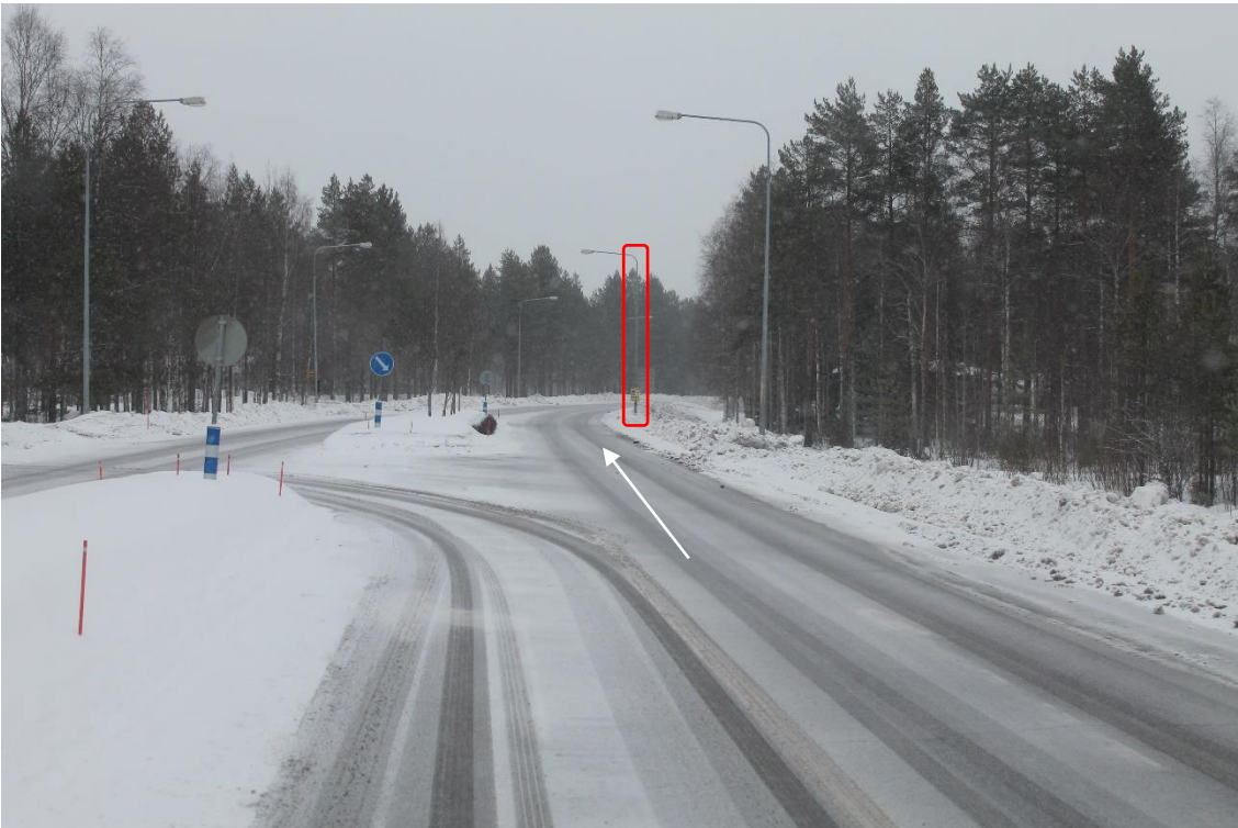
Pos 17/Pic 32. Turning from road 88 toward road 28. Marked lamp post need to be removed.
