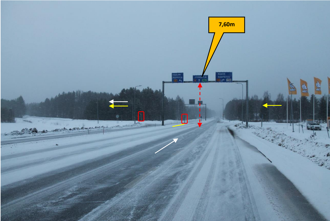
Pos 16/Pic 25. Turning from road 4 toward road 88. https://goo.gl/maps/gqsMmTAFtgPnDaHi7 Marked signs need to be removed. Marked area need to be filled. From here routes are same to site.
