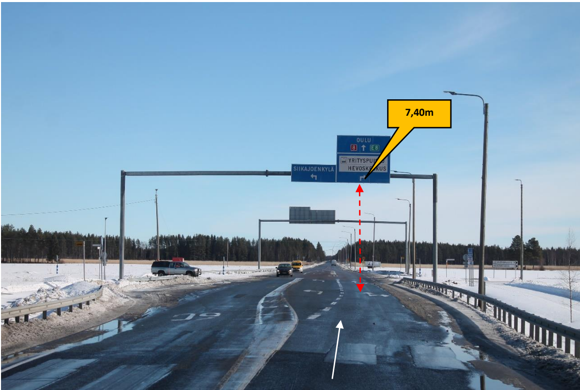
Pos 9/Pic 15. Road 8. https://goo.gl/maps/F989ccuuYAbFZHvi9 Modifications: N/A
