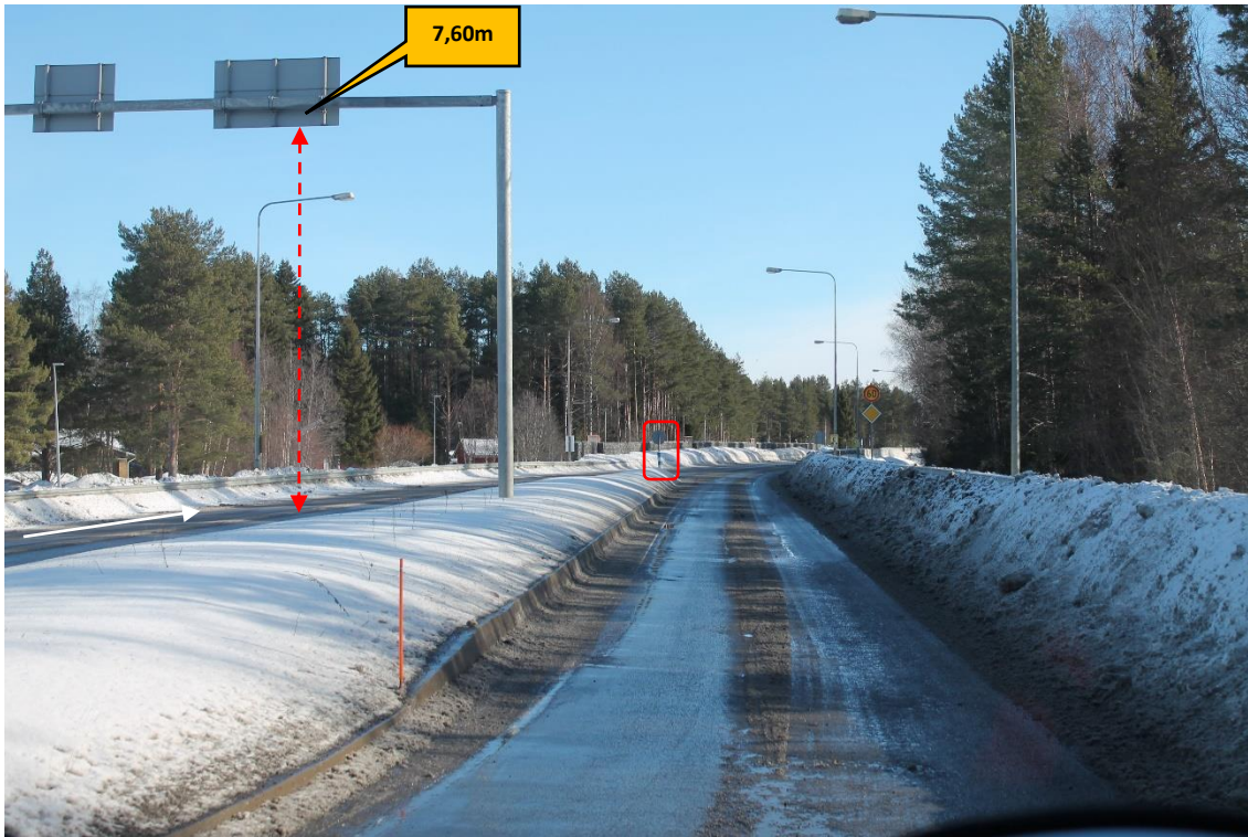
Pos 6/Pic 11. Road 8. Continue straight on counter lane. https://goo.gl/maps/zBqM1gULQySmSoFh6 . Marked sign to be removed.
