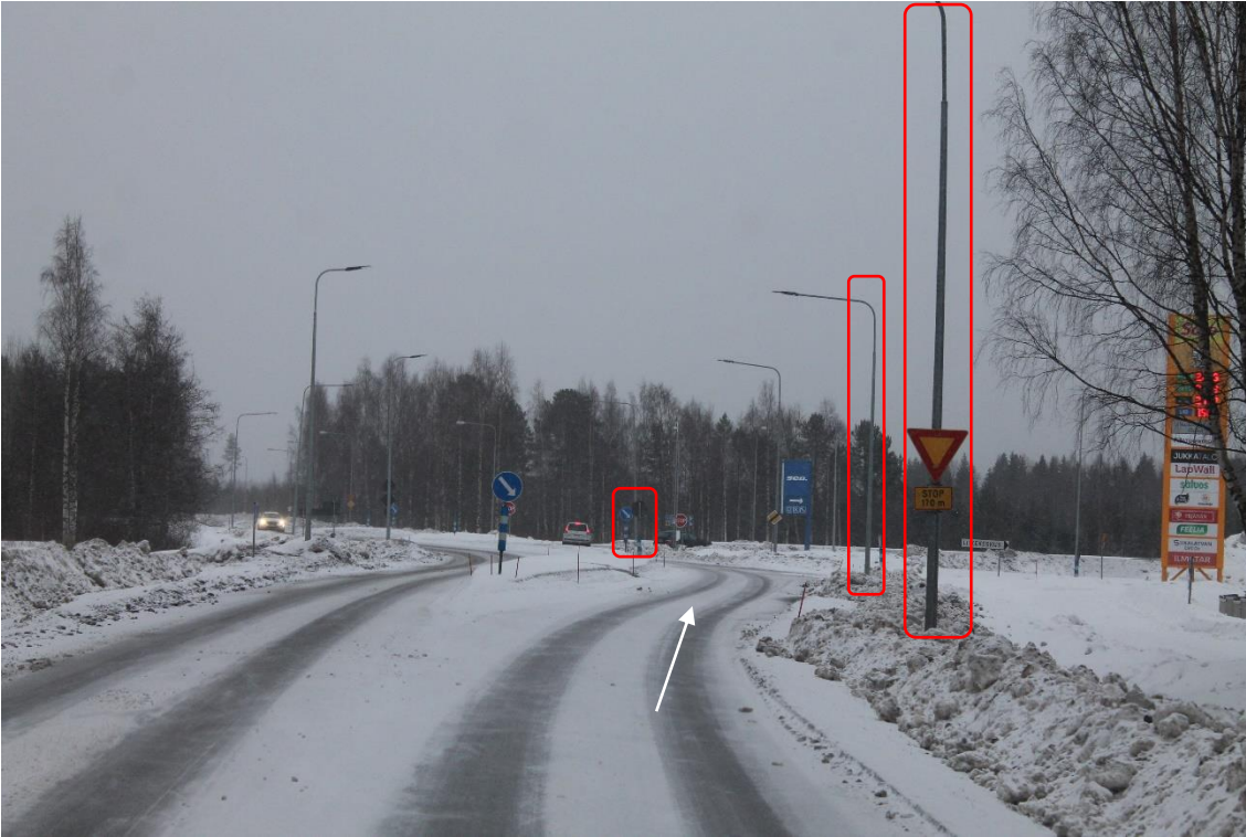
Pos 17/Pic 27. Road 88. https://goo.gl/maps/UnHpVqDEzfYUMwou7 Marked lamp posts and signs need to be removed.
