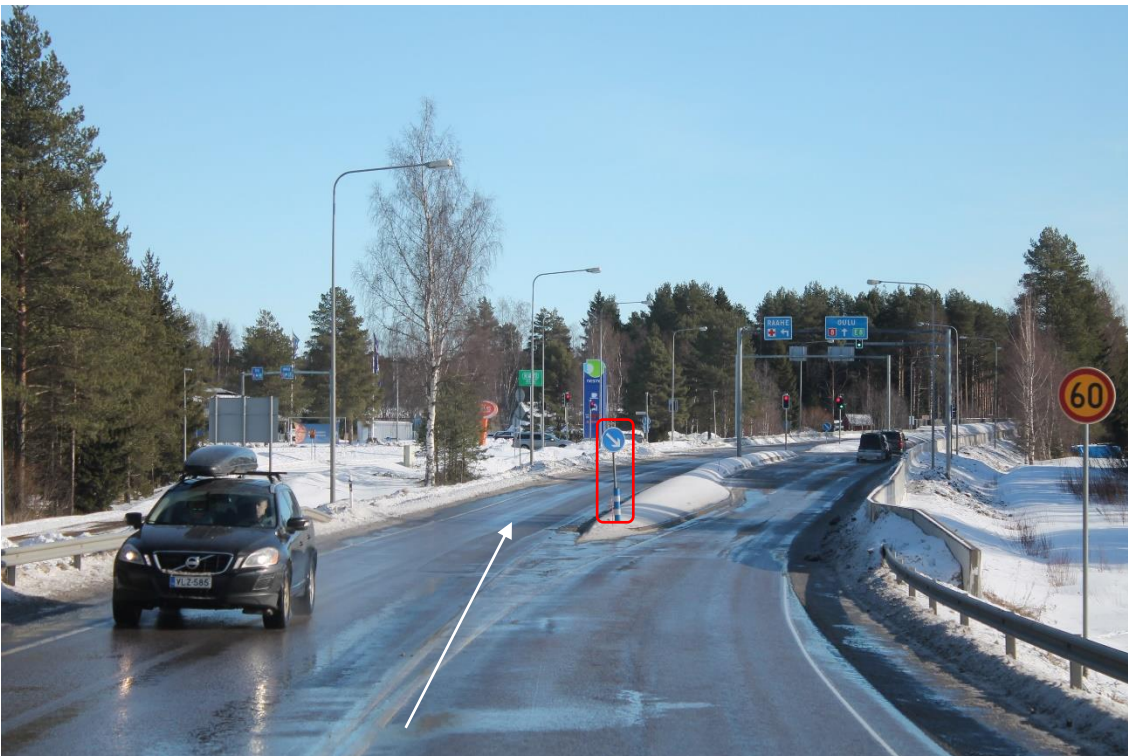
Pos 6/Pic 10. Road 8. Continue straight on counter lane. https://goo.gl/maps/zBqM1gULQySmSoFh6 . Marked sign need to be removed.
