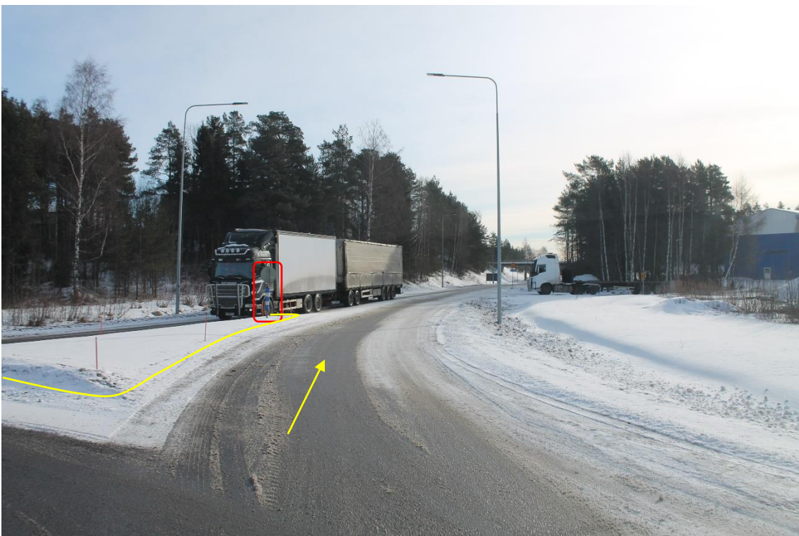
Pos 22/Pic 45. Roundabout Lapaluodontie. Marked sign need to be removed. Marked area need to be filled.
