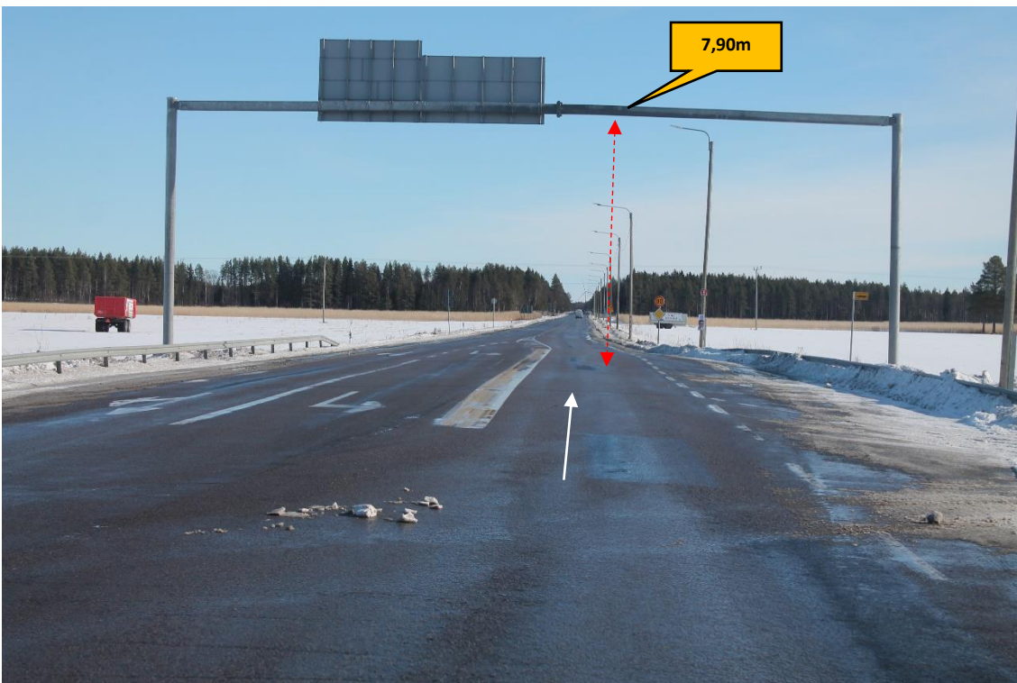
Pos 9/Pic 16. Road 8. https://goo.gl/maps/F989ccuuYAbFZHvi9 Modifications: N/A
