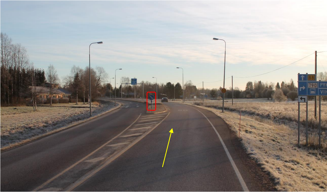
Pos 24/Pic 48. Road 88. https://goo.gl/maps/9j58sMbdbnfWDuyP9 Marked sign need to be removed.
