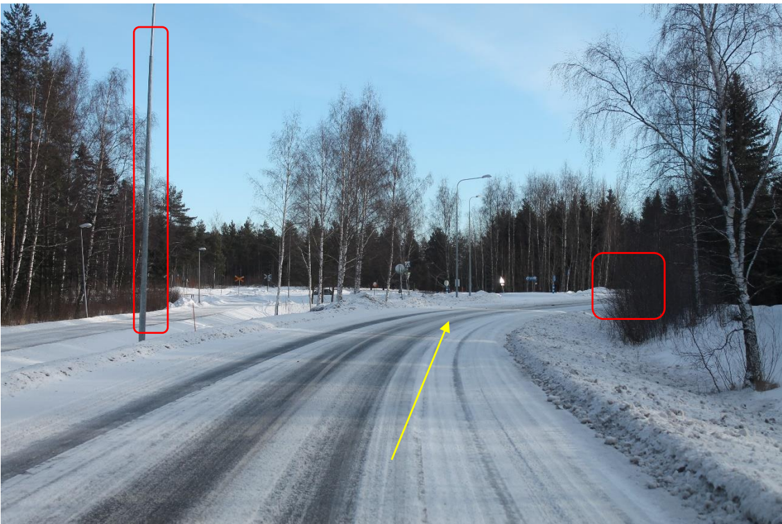
Pos 21/Pic 41. Lapaluodontie. https://goo.gl/maps/SZSvDUusUGcyWNCj8 . Marked lamp post and sign to be removed. Marked bush/trees need to cut.
