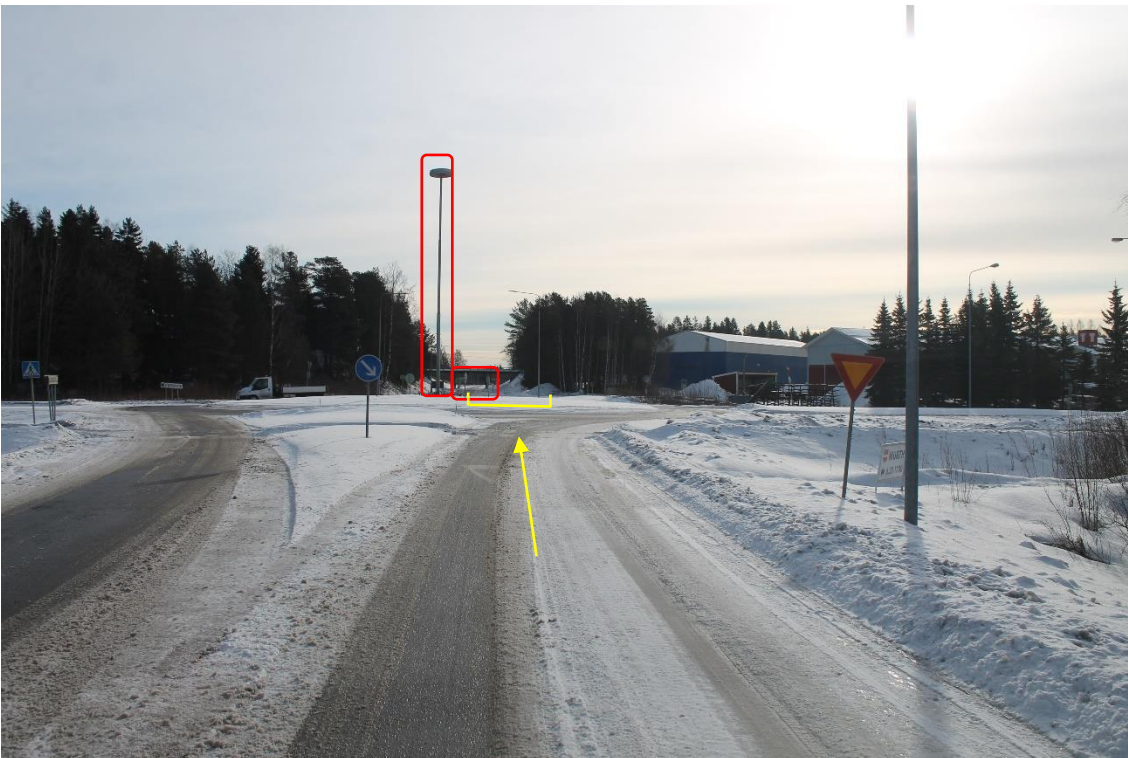
Pos 22/Pic 43. Roundabout Lapaluodontie. https://goo.gl/maps/fNoSyewtX85WBptj7 . Marked lamp post and signs to be removed. Marked area need to be filled and drivable.
